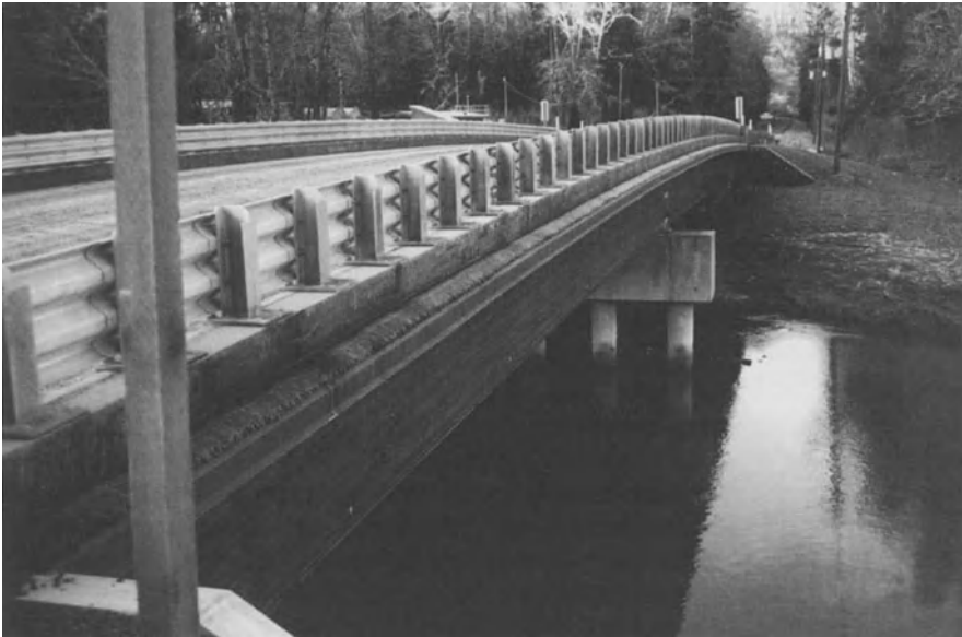
Fig. 6.7. Use of FRP glulam on Clallam Bridge, Sekiu, WA
