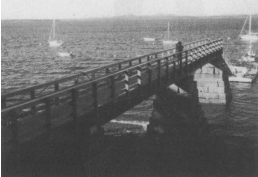
Fig. 6.88. Bridge at Bar Harbor, ME with FRP/glulam
