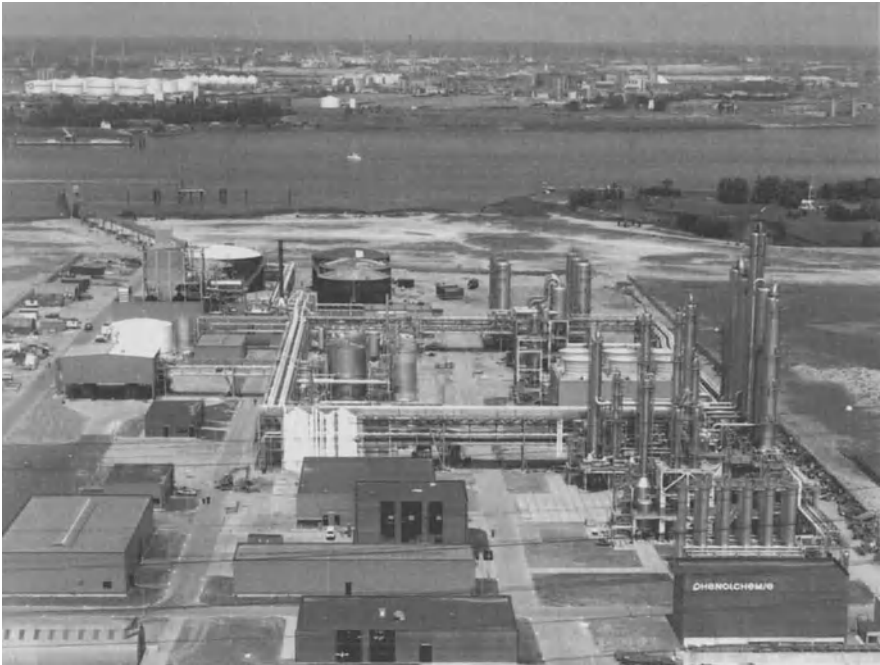
Fig. 1.2. Phenolchemie's new 200,000 tonnes per year phenol plant in Antwerp, which came on-stream in 1993
