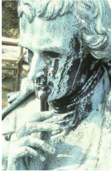
Fig. 1.5 Details of the statue of Thomas Jefferson from the Washington Monument (1858), by Thomas Crawford and Randolph Rogers, Virginia State Capitol, Richmond, VA, showing corrosion damage caused by industrial pollution. Photograph courtesy of Phoebe Dent Weil, Northern Light Studio, Florence, MA
