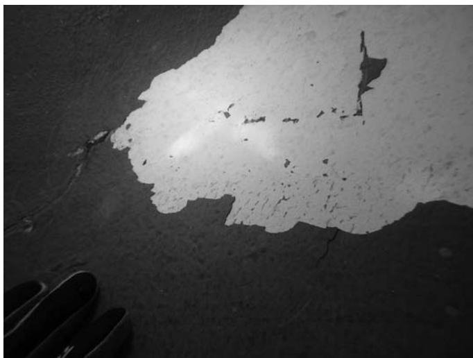
16.6 Antifouling topcoat delamination detected during an underwater inspection.
